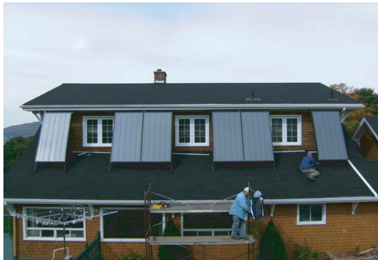
"Portrait" style Furnace Retrofit installation Roof mount
